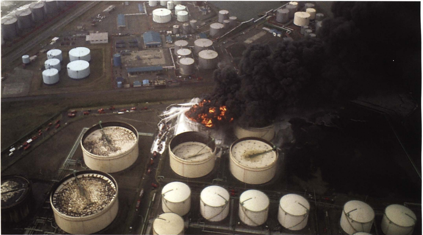
▲ Figure 1. Aerial view of the fire in the oil tank damaged by long-period ground motions from the 2003 Tokachi-oki, Japan earthquake (courtesy of Dr. Hiroshi Koseki, National Research Institute of Fire and Disaster, Japan).
